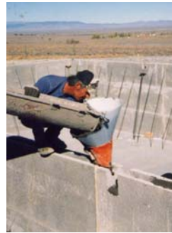
Filling the hollow wall with grout
