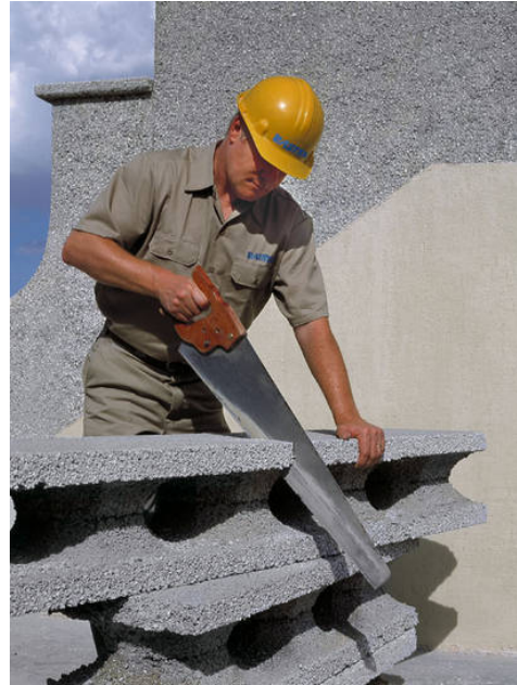
Perform Wall ICF
