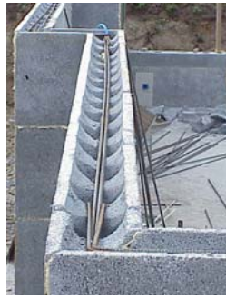
Block waiting for cement
