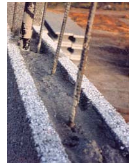
After pour is completed
